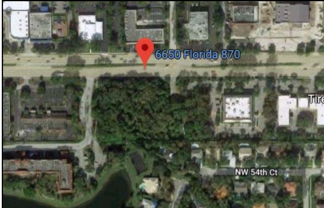
CLOSE UP AERIAL VIEW
