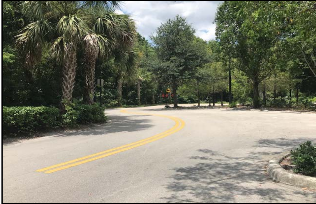
ACCESS DRIVE FACING WEST
